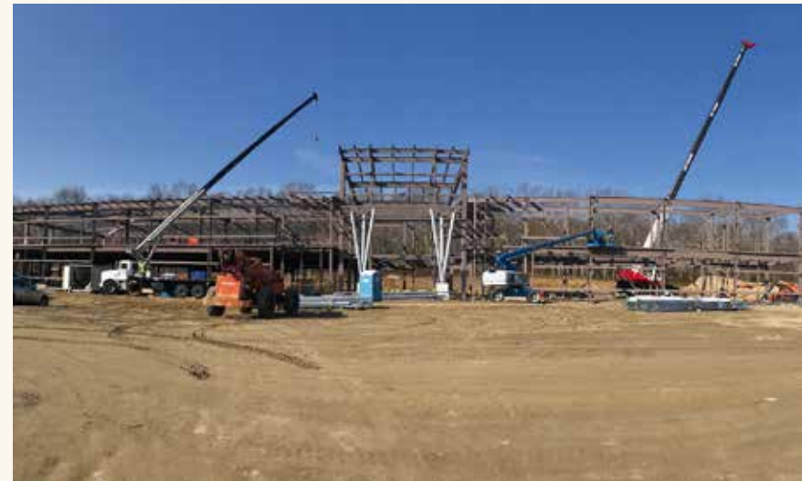
Construction of new JFHQ at Camp Fogarty
